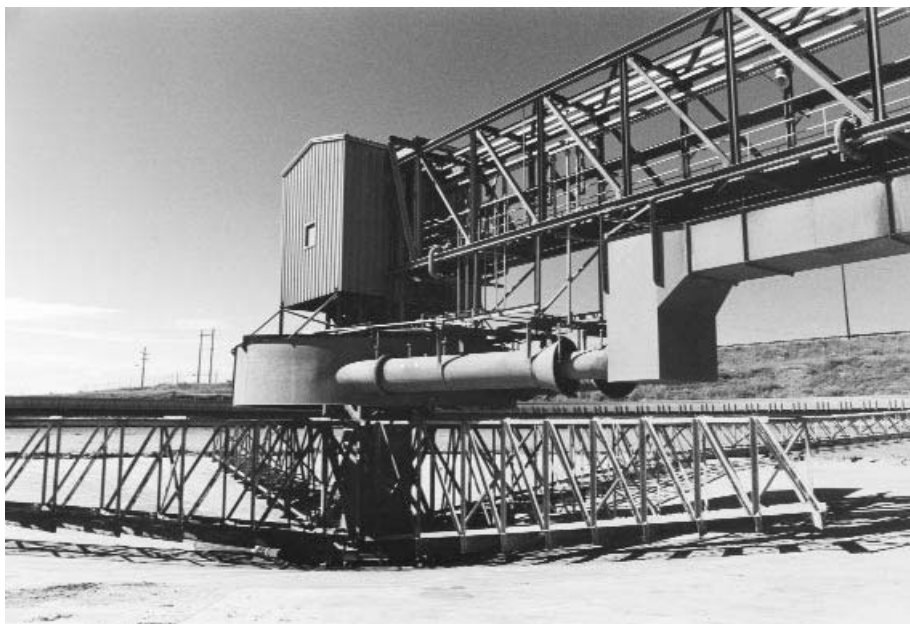
FIG. 18-92 E-Duc® Feed dilution system installed on 122-m-diameter thickener. (EIMCO Process Equipment Co.)
