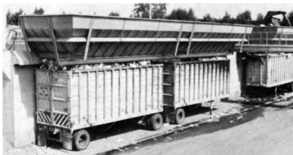
FIG. 25-62 Direct-discharge transfer station with open-top trailers located in a depressed ramp under the loading hoppers.
